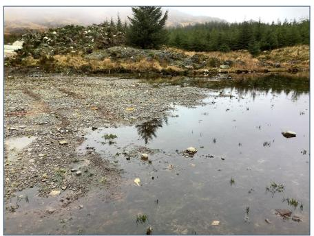
Plate 13-11: Location of proposed temporary construction compound looking N, note area already developed with peat removed.
